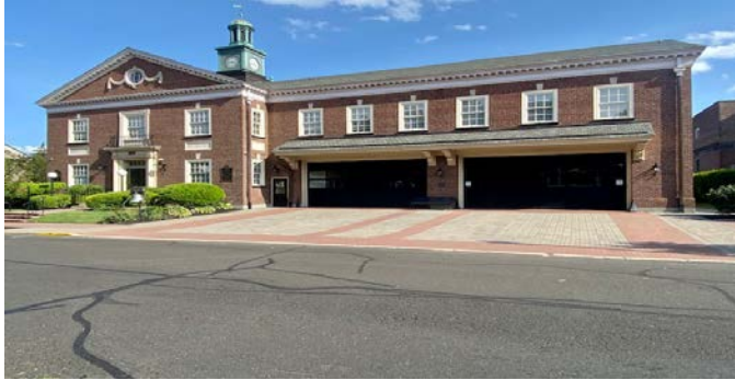
STATION 50 250 Pond Street Bristol, PA 19007 Owner Bristol Borough Year Built/Renovations 1927/2009
