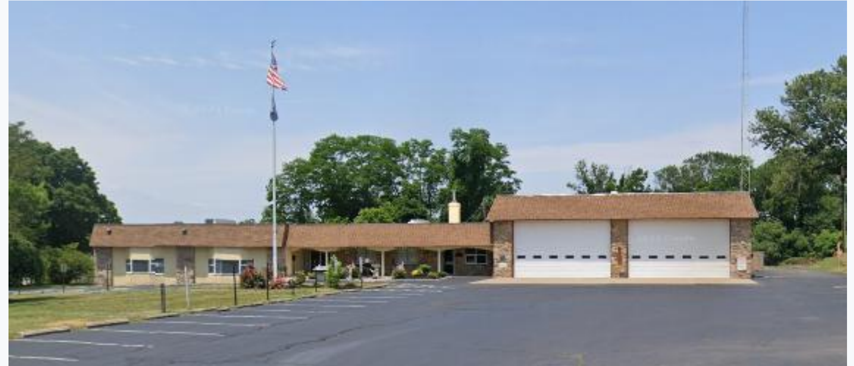
STATION 12 New Falls Road Inactive Since 2019
